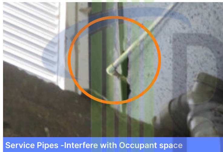
Service Pipes - Compromised envelope
