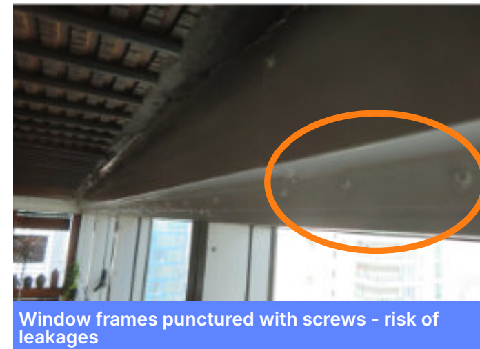
Framings damaged due to interior fixings, lead to water leakages
